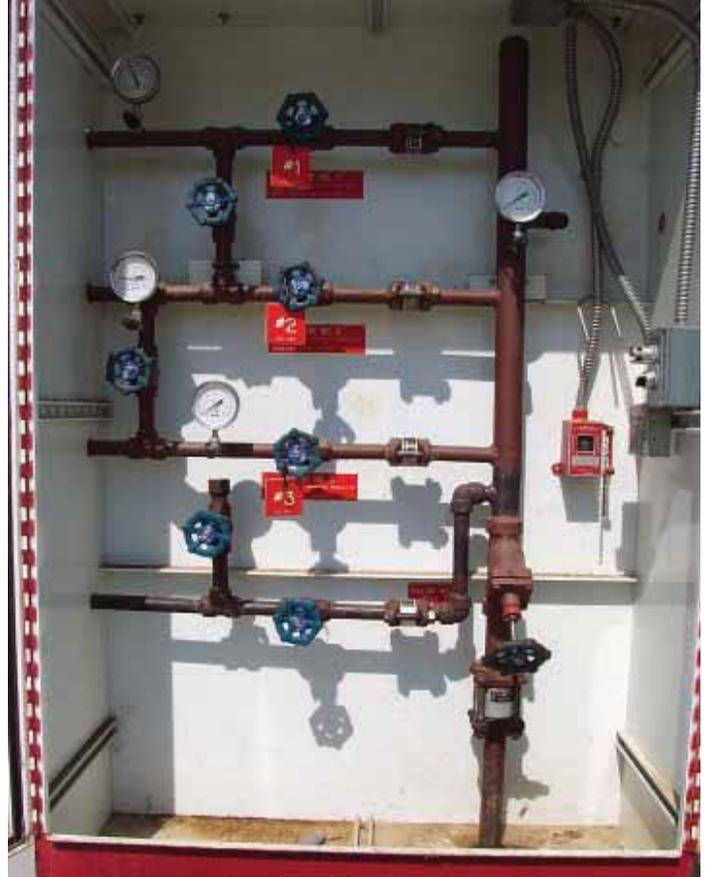
Interior of an emergency control box for an ammonia refrigeration system.
