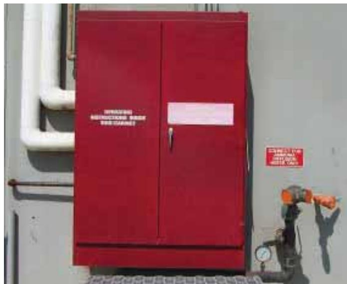
Enhancements in refrigeration system control equipment associated with new technologies now make it possible to provide an automatic emergency control system to replace key functions of the traditional manual emergency control box, like the one shown above. Such automatic controls, now required by fire codes, have made manual emergency control boxes obsolete.
