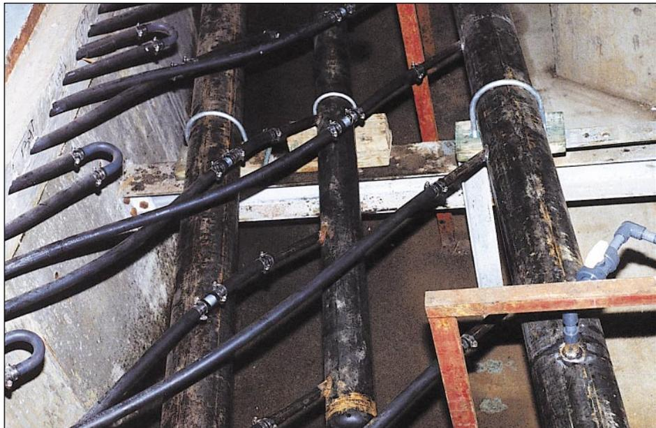
**The large number of joints in the 1-in. polyethylene pipe are due to the demolition subcontractor's cutting them all short before reading the specification.**
